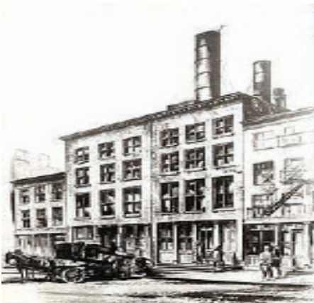
POWER PLANT 1882 PEARL STREET STATION
