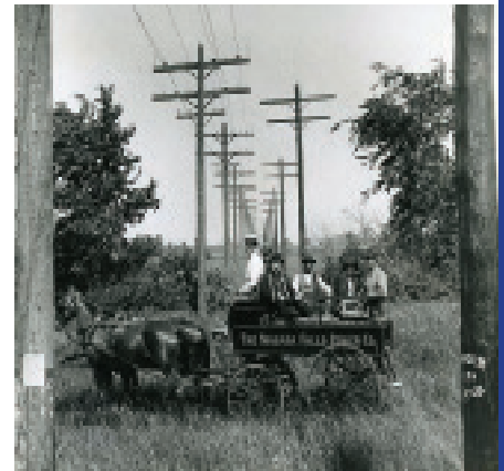
TRANSMISSION LINES 1902 NYAGARA POWER CORPORATION(11KV)
